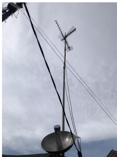
Figure 9. Implementation of the 433 MHz wokbolic antenna
